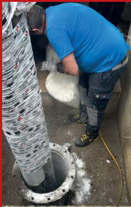
BoreSaver Ultra C is poured into the borehole of a well in Italy that had all but been mothballed due to problems with bacteria dramatically reducing its output
