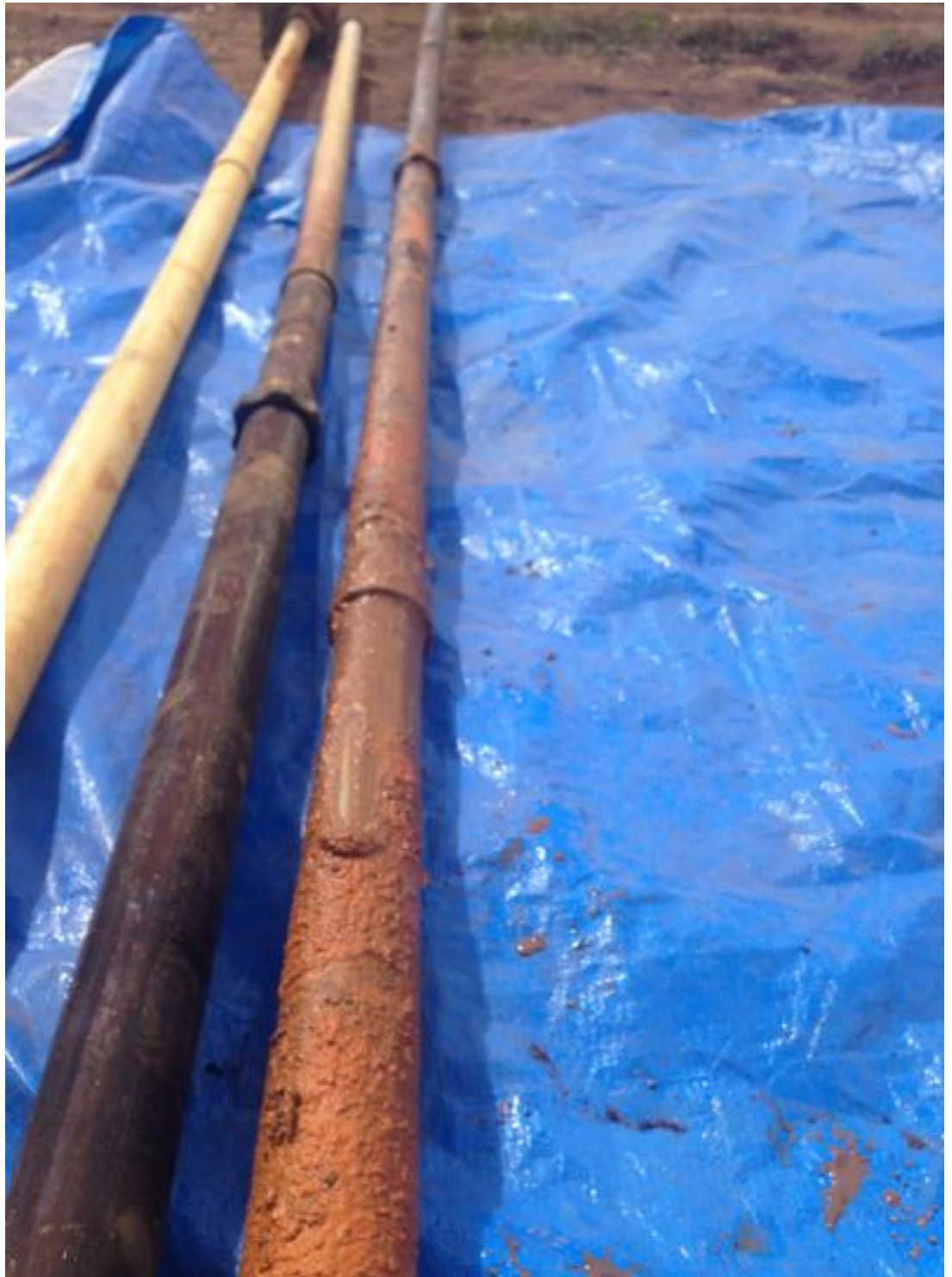
Progression on the rising main from a clean pipe at the top, to black precipitates and the orange Fe-oxide precipitates and slime (Credit: Jamie Rattray)
