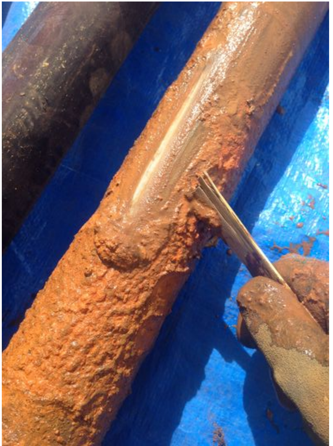
The extent of the slime on the rising main after it was removed as part of the wellbore forensics programme (Credit: Jamie Rattray)
