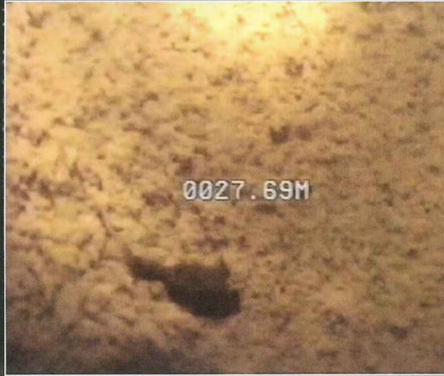
Left to right: removing the pump from the G150 well in the Gwelup Borefield; G140 Well in the Gwelup Borefield. A side view picture of the Johnson wedge wire wound well screen, 27m down, prior to cleaning. The screen is almost completely obscured by soft, slimy biofilm and residue caused by iron bacteria; the same screen after treatment but at a depth of 43m
