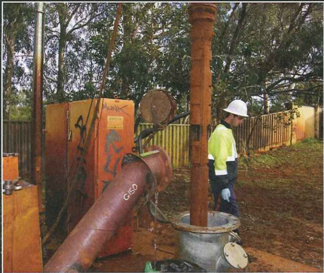
Left to right: removing the pump from the G150 well in the Gwelup Borefield; G140 Well in the Gwelup Borefield. A side view picture of the Johnson wedge wire wound well screen, 27m down, prior to cleaning. The screen is almost completely obscured by soft, slimy biofilm and residue caused by iron bacteria; the same screen after treatment but at a depth of 43m
